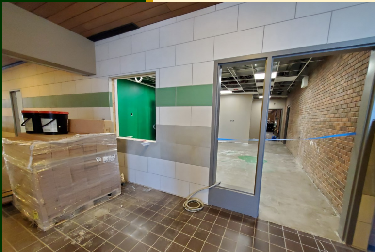
The Main Office, above, is the secure point of entry for the building. Visitors must go to the reception window to be buzzed into the locked interior foyer doors, or to be buzzed into the office.
